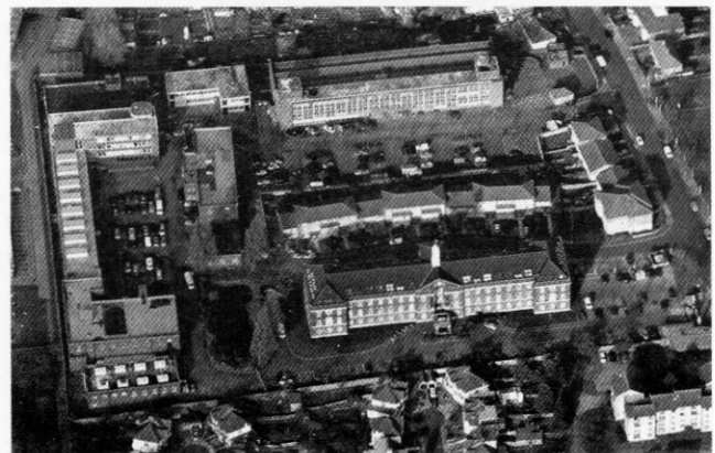
The buildings due to be demolished are on the left. Building 15 is at the top and the Paddock bunker is below the houses on the right.
